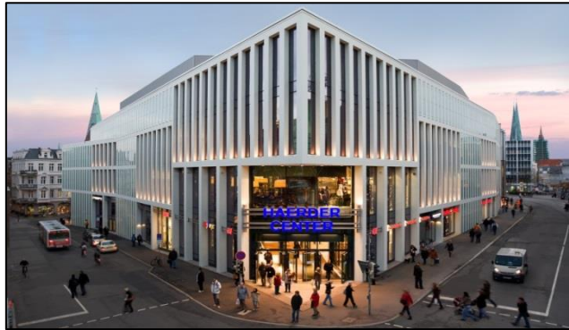
Lübeck (Haerder-Center) Sandstr. 1
