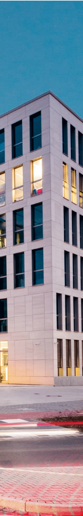
The office property Ratingen is characterized by its energy sustainable features and sets standards as a "green building"
