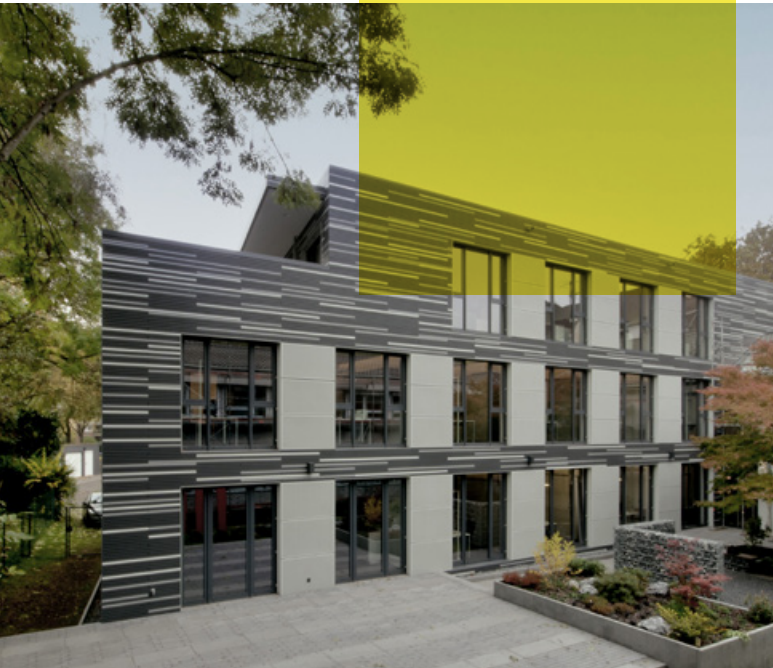
Headquarters of HAMBORNER REIT AG, Duisburg, Germany
