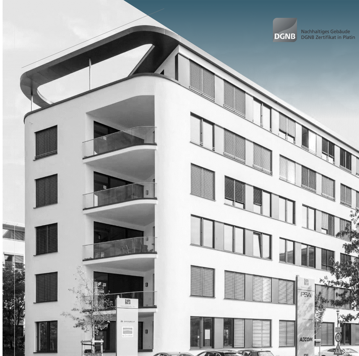
Office property Neu-Isenburg
