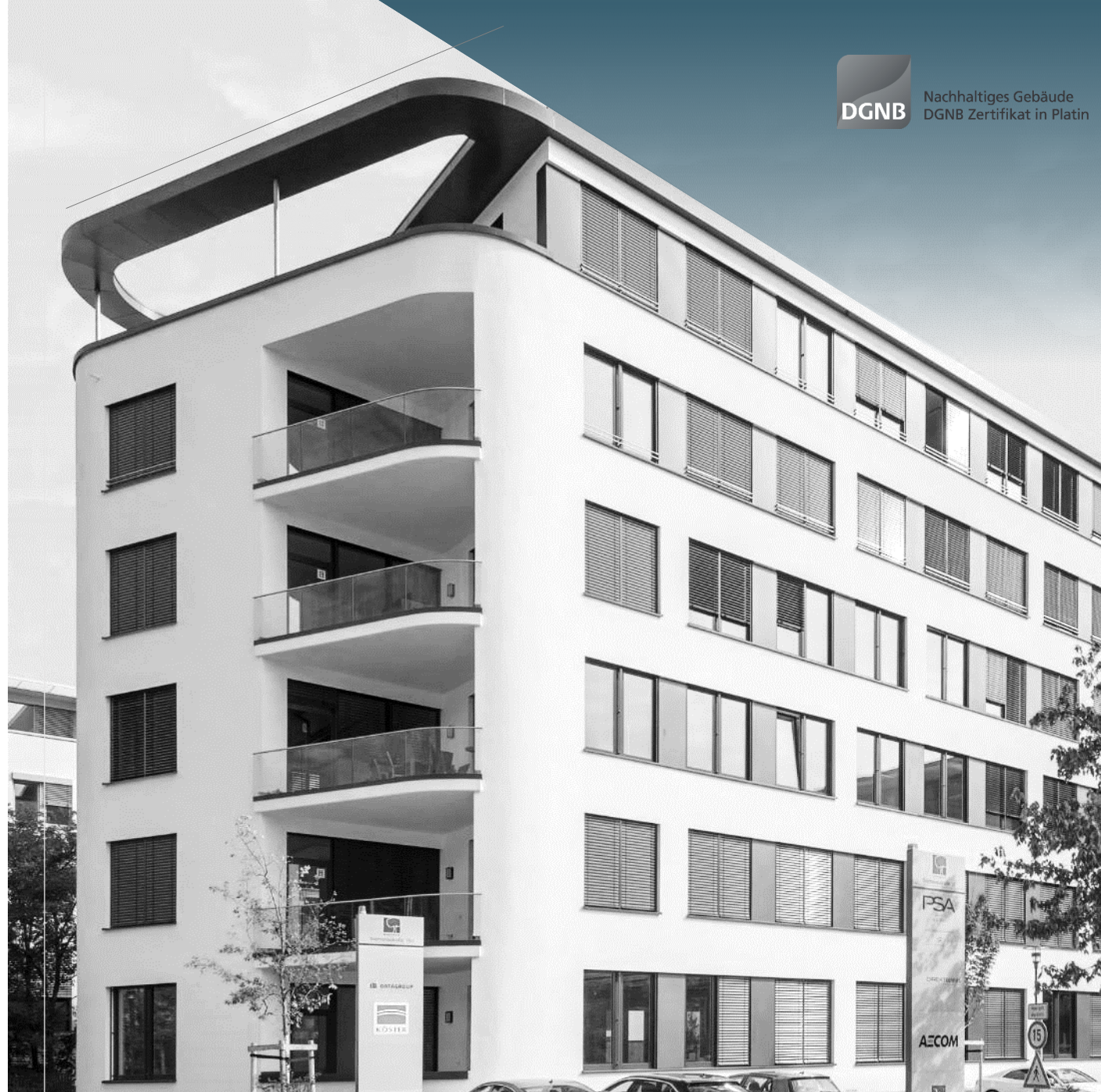
Office property Neu-Isenburg
