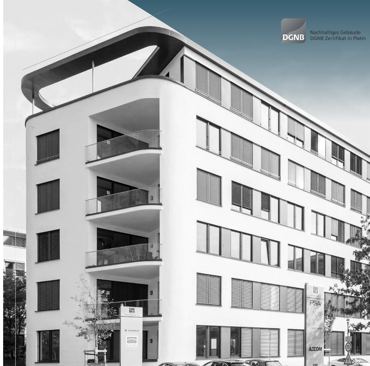
Office property Neu-Isenburg
