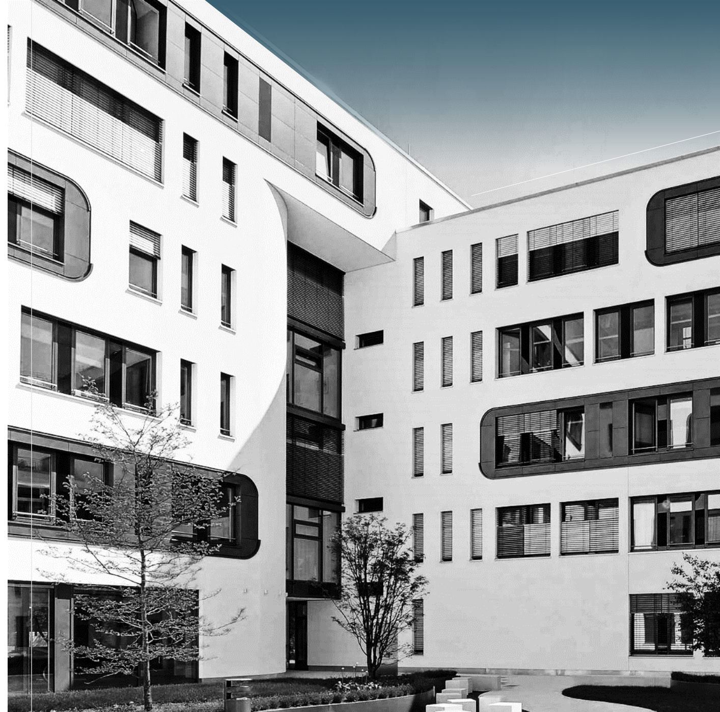
Office property 'Nu-Office' in Munich
